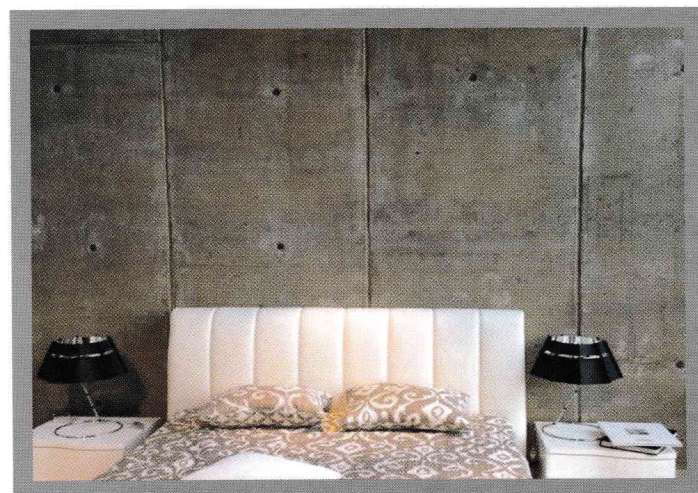
↑ Plank Joint With Screw Effect
